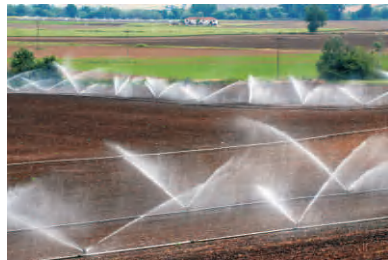
Commercial/Agricultural irrigation system
